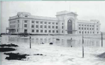
CN Rail Station, Archives; 1917
